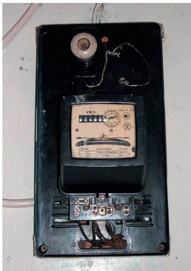
Picture 2.4: Individual billing is not possible since the installed electricity meters do not function properly. (Photo: T. Hoeck, June 2003)
