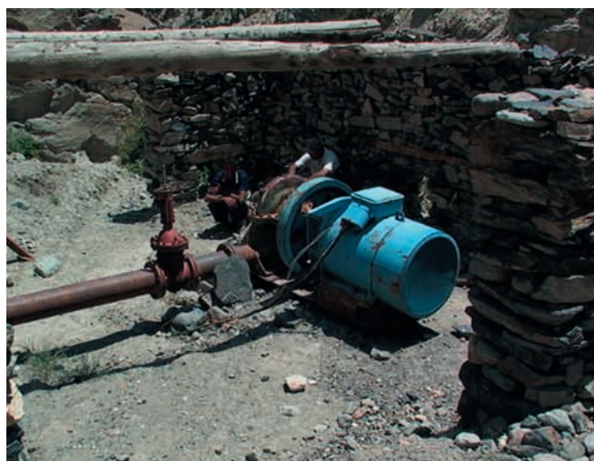
Picture 2.11: Due to antiquated equipment and lack of know-how to perform repairs, the MHPS in Roshorv has not been operating since October 1998. (Photo: R. Droux, July 2003)
