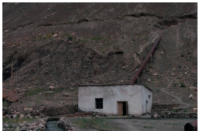
Picture 2.15: Water channel and leaking forebay tanks cause erosion and reduce water supply for the hydro scheme. (Photo: T. Hoeck, June 2003)
